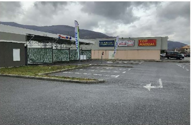
Photo 22 Station service Source: LIDL
