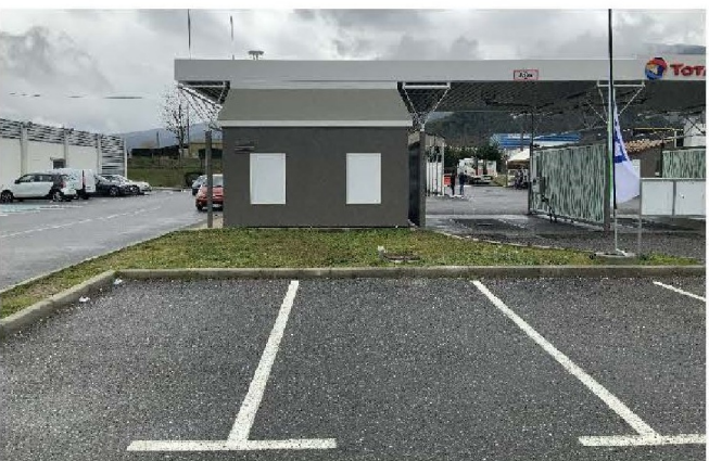
Photo 21 Station service Source: LIDL
