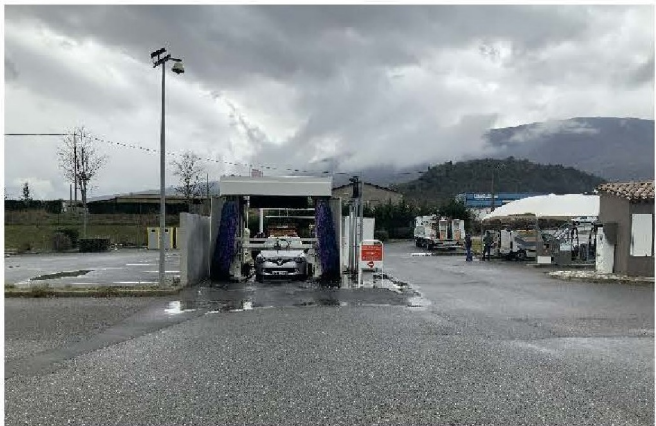
Photo 20 Station service Source: LIDL
