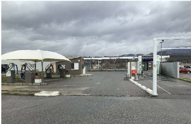
Photo 18 Station service Source: LIDL
