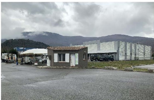
Photo 19 Station service Source: LIDL
